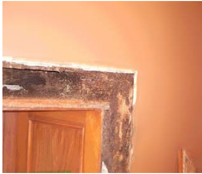
Fig 1a. Visible image of door jam, no evidence of termite infestation
